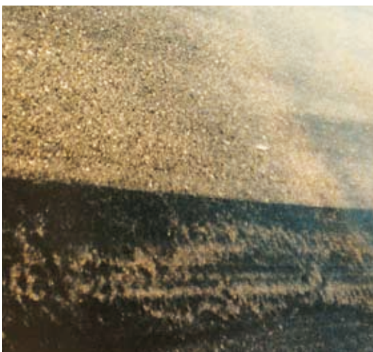
Rubber removal from airport runways upper: after cleaning lower: uncleaned (Efficiency up to 1,500 m 2 /h)
