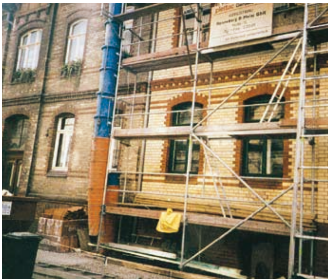
Brick facade, cleaned by waterjetting
